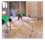
Moisture Barrier. Place & level a layer of granular fill. Place a 6-mil polyethylene moisture barrier over the granular fill.
